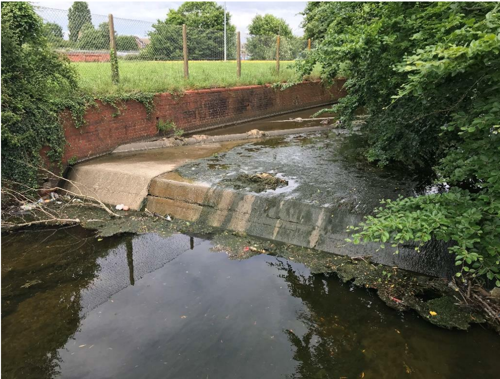
Graphic 3-3 The most upstream of the sequence of step weirs within Hermitage Stream (photo taken looking upstream)
