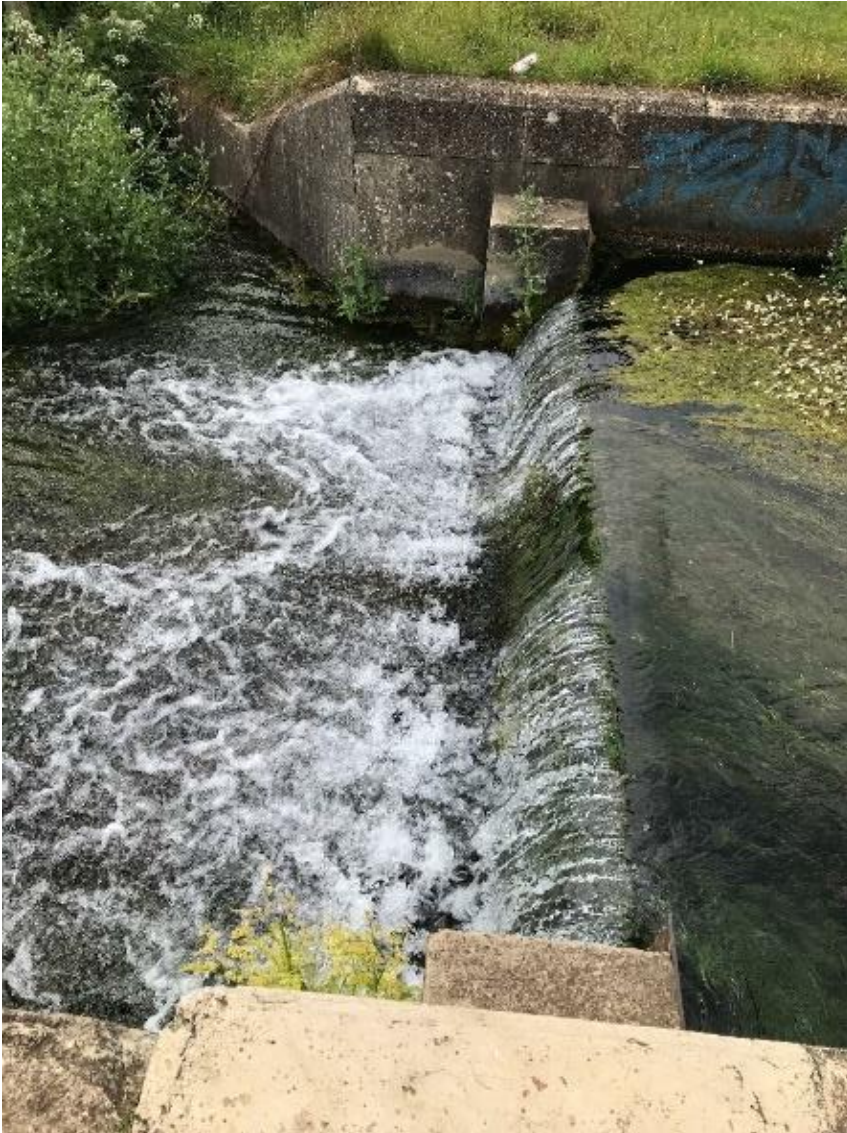
Graphic 3-5 Single vertical faced weir within Hermitage Stream
